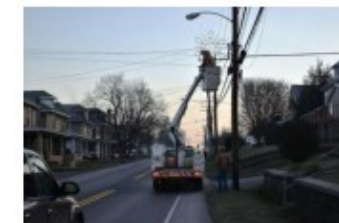
Lights installed on the pole
